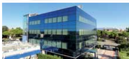
ROVER Laboratories and offices
